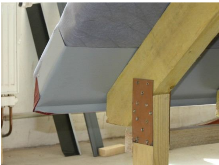
Breathable water resistant underlay – RIDGE nonventilated attic space of height > 1,5 m
