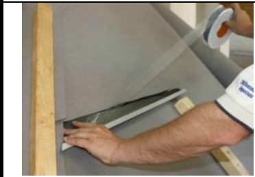
4.4 stick membrane on drainage ditch with tape JTD SP 38
