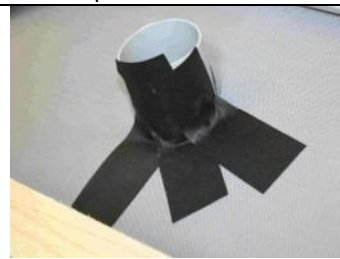
4.12 - 4.13 use the tape JUTADACH SP SUPER to seal the circular penetration – start at the bottom and continue upwards
