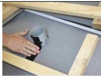
4.12 - 4.13 use the tape JUTADACH SP SUPER to seal the circular penetration – start at the bottom and continue upwards
