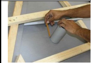
4.8 retrace the circular penetration on the membrane
