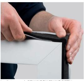
Installation example ISO3-WINDOW SEALING SYSTEM
